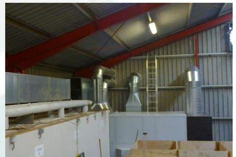
Air duct connected to new adsorption air dryer.
