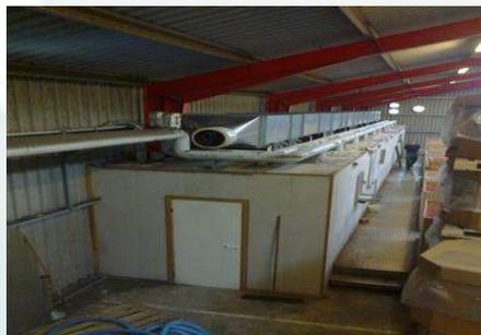
New air duct on plenum to distribute dried air per section.
