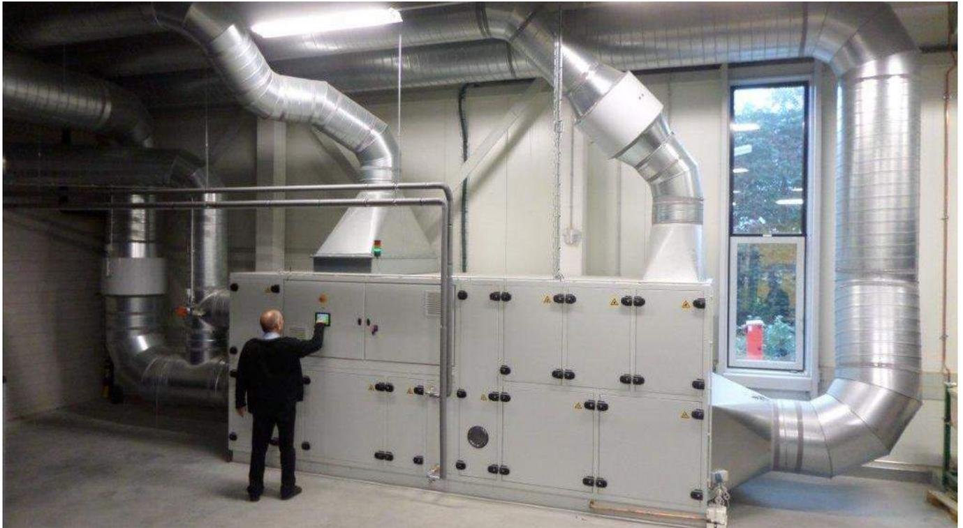
Dehydrated air by absorption or special Hybrid dryers.
