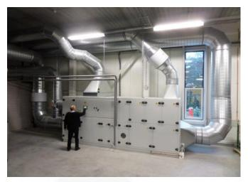
Agratechniek has developed a principle at which a **central air dryer (1)** brings the dried air to where it is needed **(1A)**. Various drying installations **(4, 5)**, Cabinet dryers (static **(6)** and rotary **(7)**), conditioning cells **(2)**, drying tables **(3)** or packing machines **(8,9)** are connected to a central air duct **(1A)**. Thanks to the advanced ABC process the dried air is discharged automatically to where it is needed at that moment.
